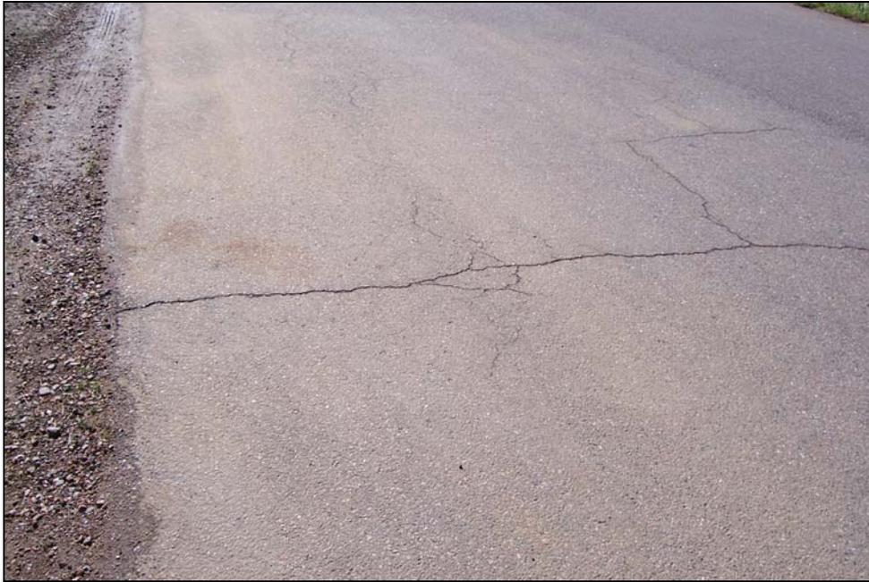
**FIGURE 11: Medium Severity Transverse Cracking**
