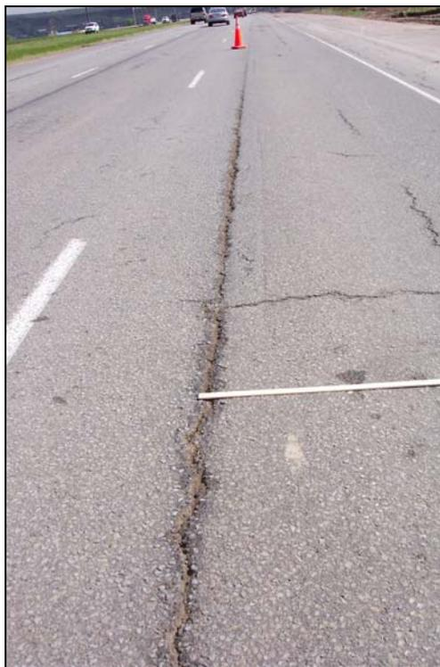
**FIGURE 7: High Severity Longitudinal Cracking**
