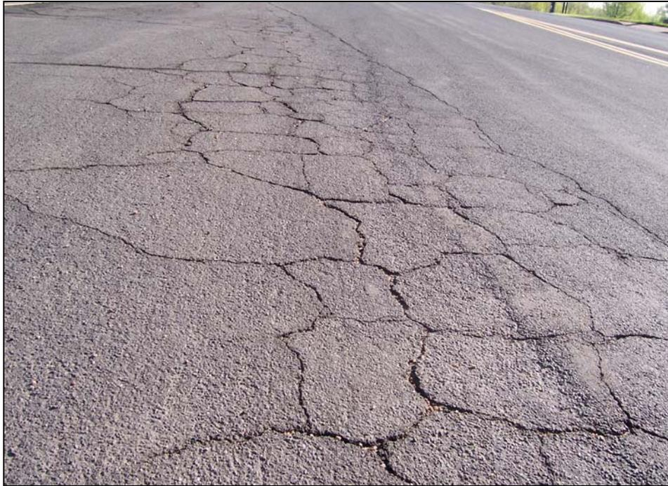
**FIGURE 5: Medium Severity Alligator Cracking**
