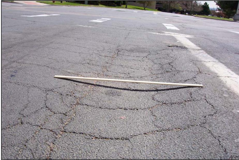
**FIGURE 19: High Severity Rutting**
