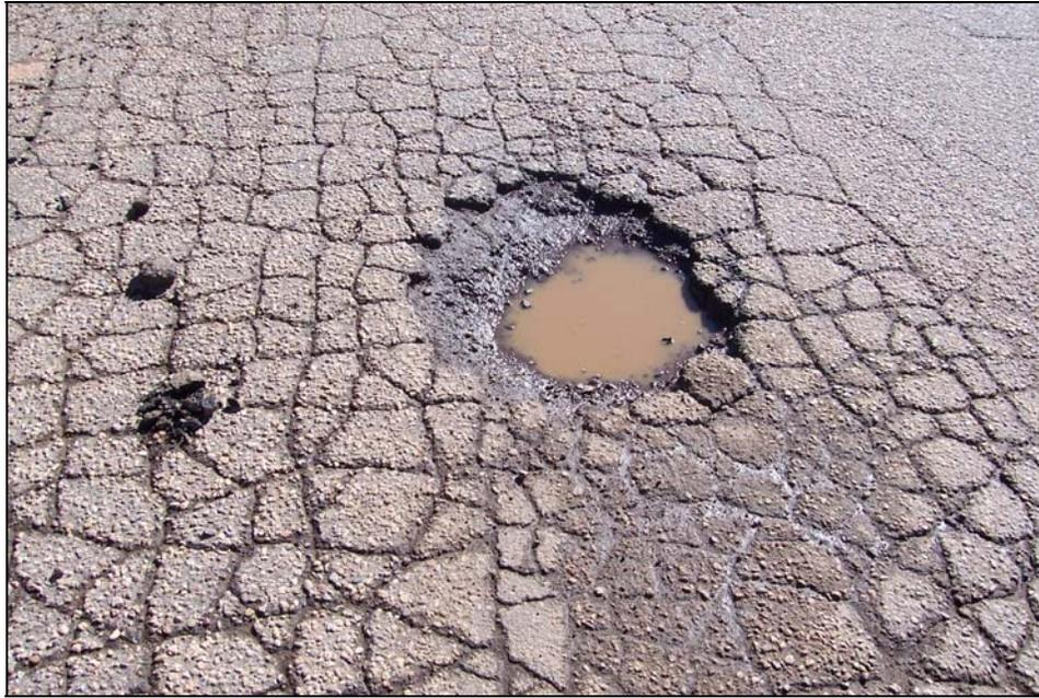
**FIGURE 16: Pothole Surrounded by Alligator Cracking**
