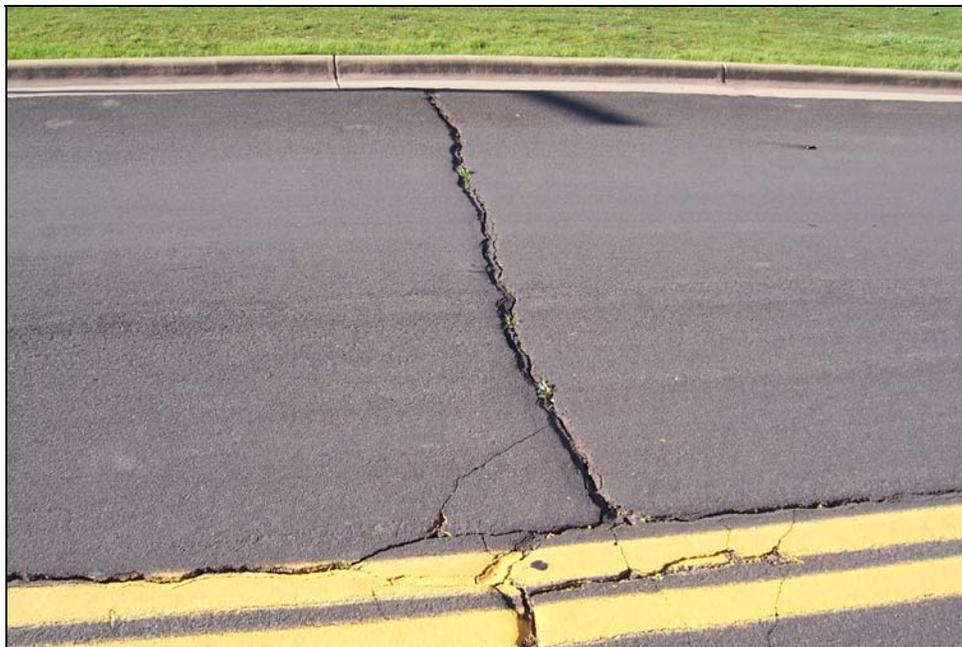
**FIGURE 10: High Severity Transverse Cracking**
