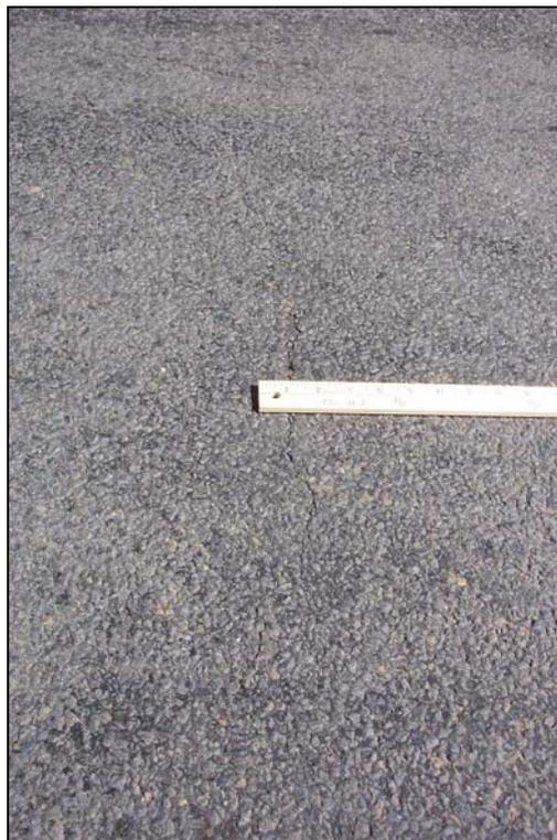
**FIGURE 12: Low Severity Transverse Cracking**
