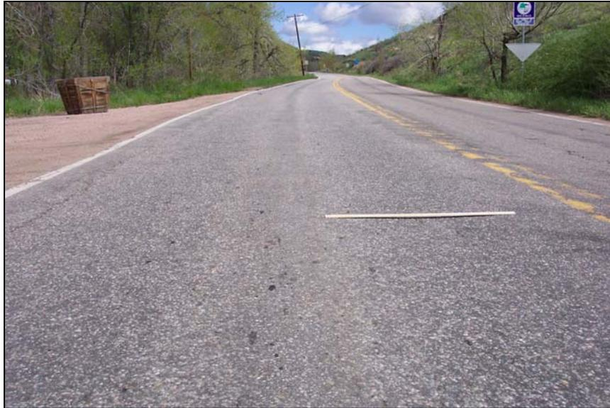
**FIGURE 21: Low Severity Rutting**
