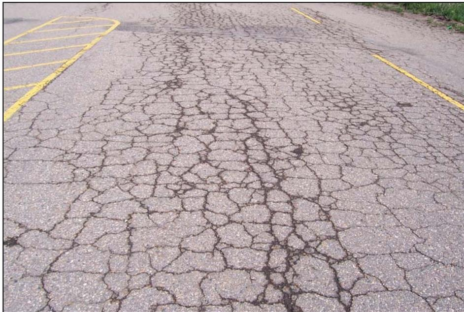
**FIGURE 4: High Severity Alligator Cracking**
