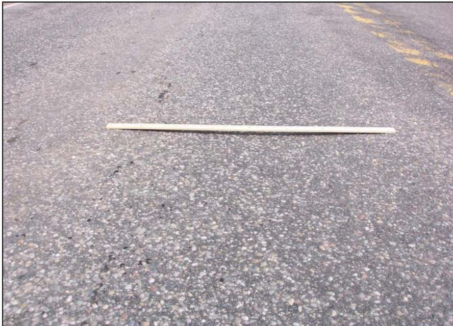
**FIGURE 20: Medium Severity Rutting**
