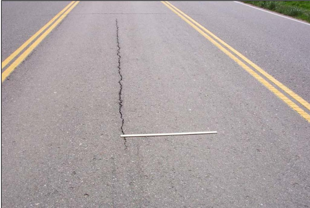
**FIGURE 8: Medium Severity Longitudinal Cracking**
