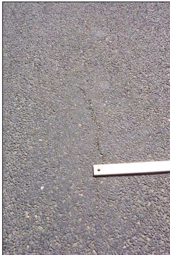
**FIGURE 9: Low Severity Longitudinal Cracking**
