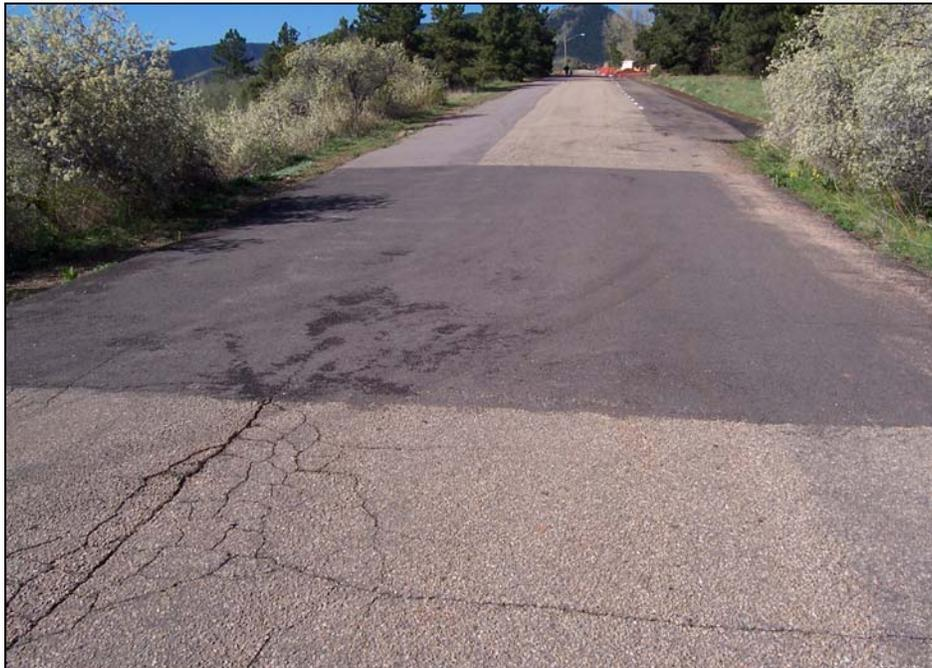
**FIGURE 17: Full and Partial-Width Road Patching**
